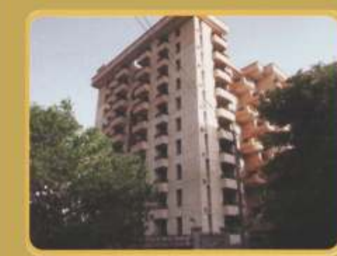
Khattar Co-operative Apartments Consisting 100 units
